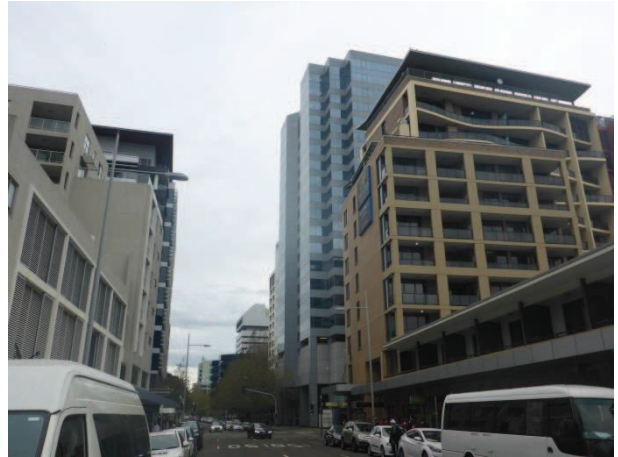
PICTURE 2 – VIEW OF THE SUBJECT SITE AND SURROUNDING DEVELOPMENT FACING WEST ALONG GEORGE STREET ('HARRISFORD' IS TO THE RIGHT OF FRAME, NOT VISIBLE)
