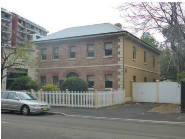
PICTURE 5 – VIEW OF THE PRINCIPAL FAÇADE OF 'HARRISFORD'
